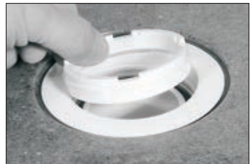
Positioning the Compression Nut
