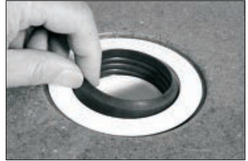
Installing the Compression Gasket
