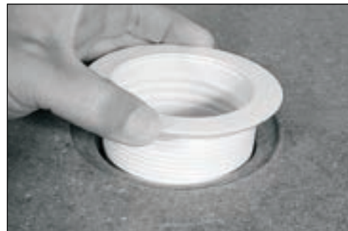
Inserting Drain Body from Top Side
