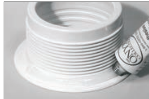
Applying Adhesive to Flange
