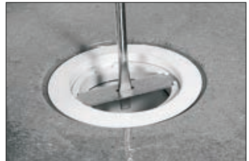
Tightening the Compression Nut
