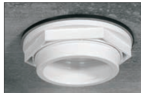
Drain Body Installed - View from Bottom
